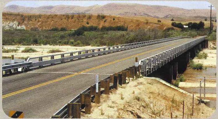
OUR LARGEST BRIDGE, 15 MATCHING RAILSPAN® MODULES WITH RAILING, 400' X 25'.
