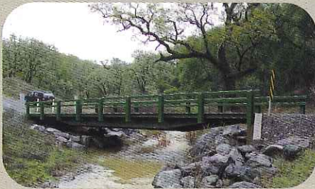
RURAL COUNTY ROAD BRIDGE.
