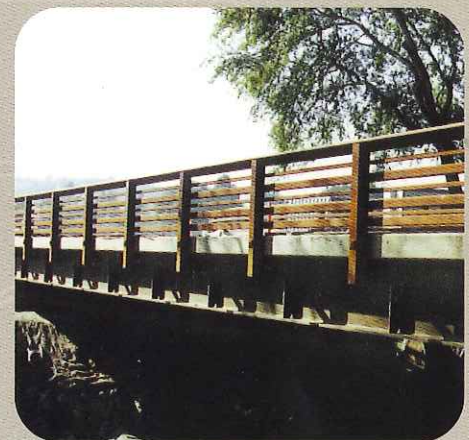
SIMPLE ARCHITECTURAL LINES OF SIDEVIEW OF SUBDIVISION BRIDGE.
