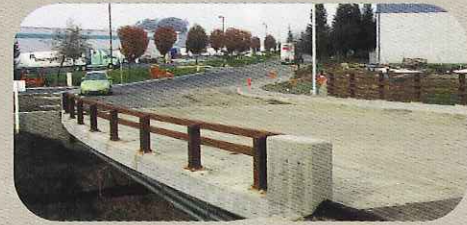
INDUSTRIAL PARK ENTRANCE BRIDGE.
